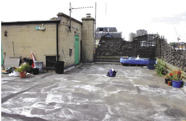
The existing asphalt roof at the FOE headquarters in London.
