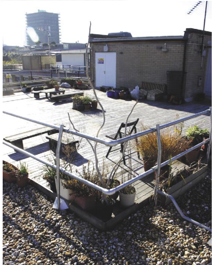
The finished roof with leisure terrace area and gravelled drainage area.
