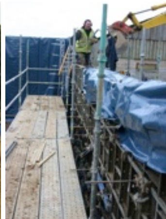
7. Shuttering protected against rain. Independent scaffolding.
