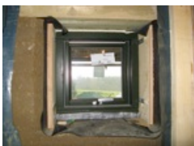
13. Small window in ply lining on DPC
