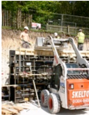
5. Chalk being delivered to shutter by Bob-cat
