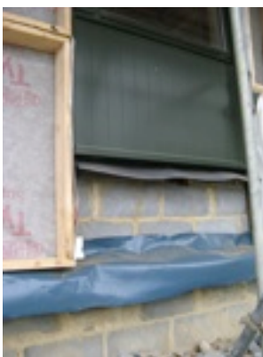
11. Ultra-light blocks used under window
