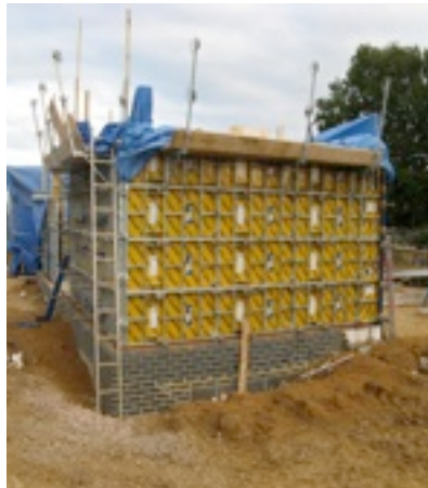
6. Shuttering with built-in access stages
